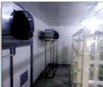
Koji room showing misting/cooling units and racks for SSF trays
