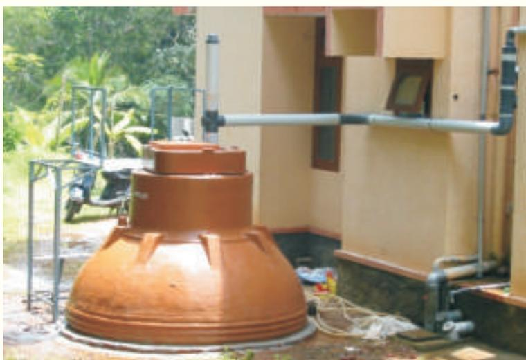
*Sewage treatment device HSD installed at an apartment*
