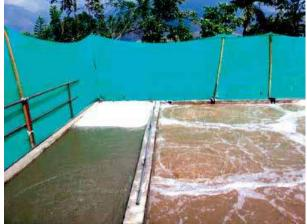
Fishmeal ETP showing an anoxic tank and one of the activated sludge tanks with submerged fine bubble diffusers
